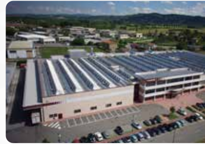
Walvoil S.p.A. Production and Logistic pole Bibbiano (RE)
